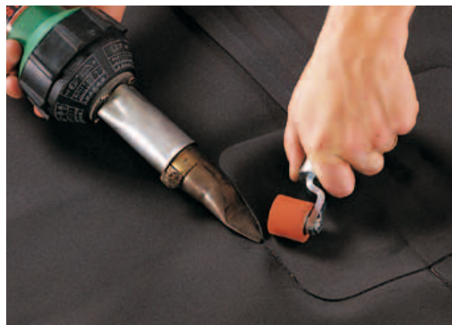
Prefabricated pipe boots, flashings and details are seamed with hot air guns. Quality control testing is provided by means of high pressure air lance testing.
