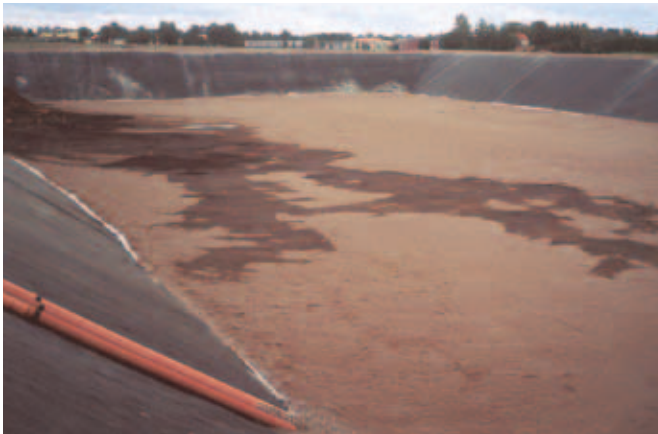
Bottom liner at landfill site, Avesta, Sweden. Owner: AvestaPolarit Contractor: Hedbergs Tak
