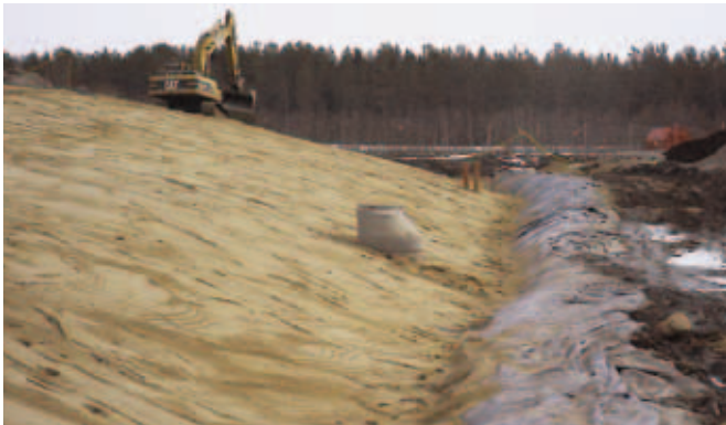
Perimeter capping at Däva industrial landfill site in Umeå, Sweden. Owner: Umeva. Contractor: Åke Larsson Grävare AB.
