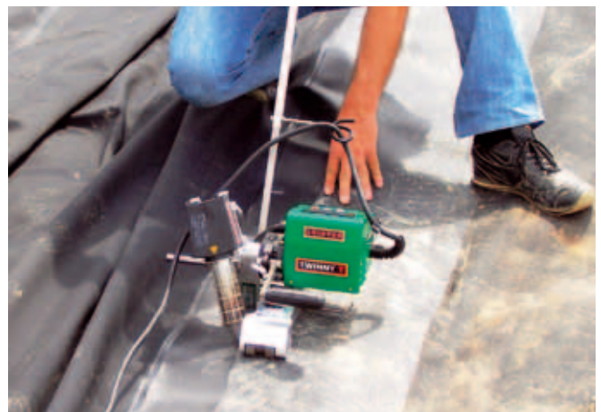
Thermal fusion seaming
